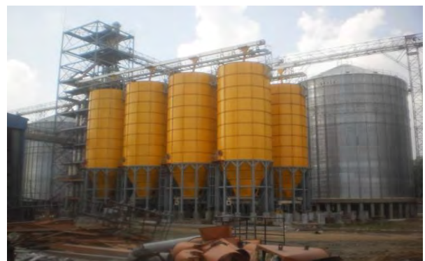
4000MT & 250MT Silo at CPChittagong Feed Mill Project, Mirsarai, Chittagong.
