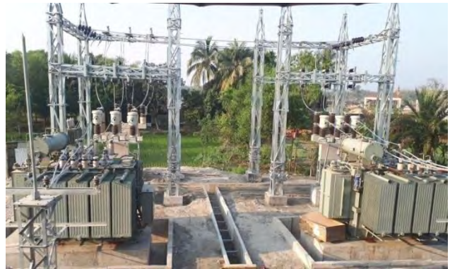
33/11 KV, 14x2 MVA AIS Sub-station at Valuka, Mymensing
