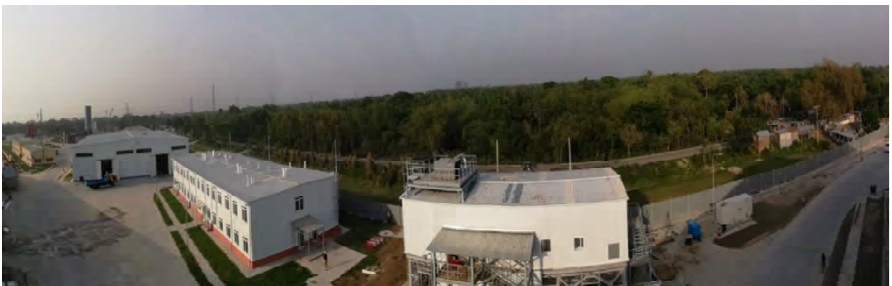
Rooppur Nuclear Power plant Project
