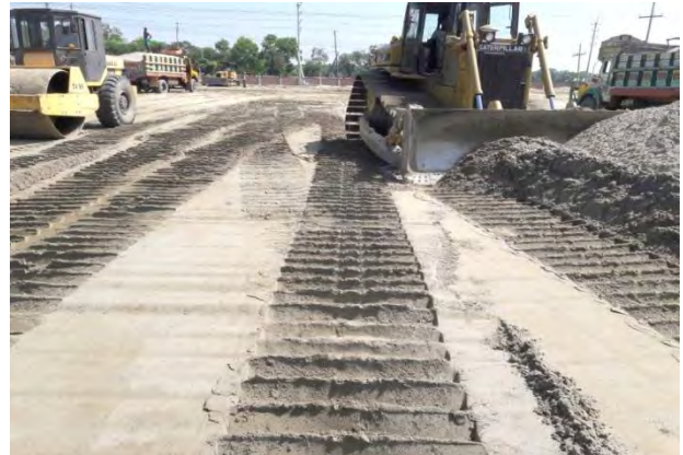
Land Filling work at Trishal Feed Mill Project
