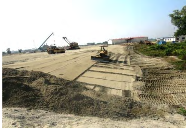
Land Filling work at BATB Savar Land Fill Project
