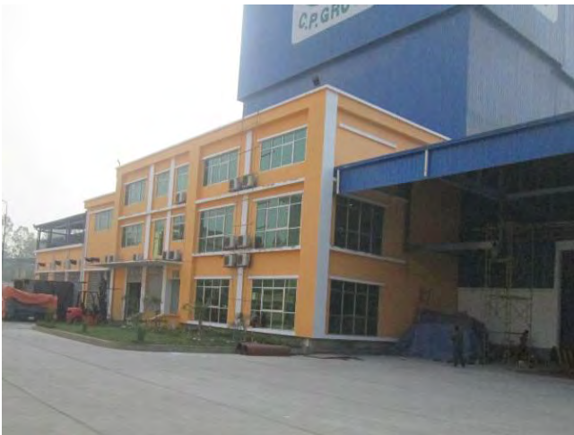
3 Storied Production Building, Total Area: 1950 sqm at C.P Chittagong Feed mill Project, Chittagong.
