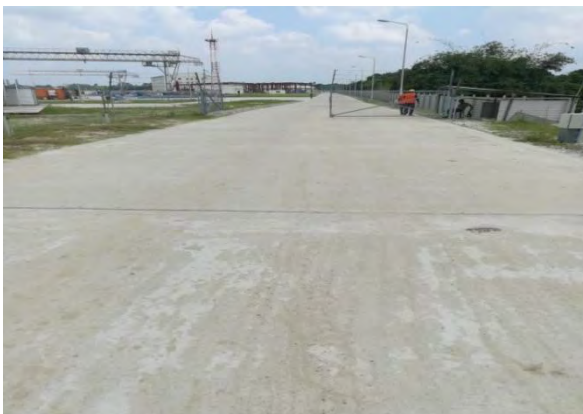
Internal Road/Pavement work at Rooppur NPP Project
