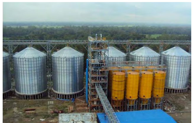
4000MT & 250MT Silo at CP Chittagong Feed Mill Project, Mirsarai, Chittagong.
