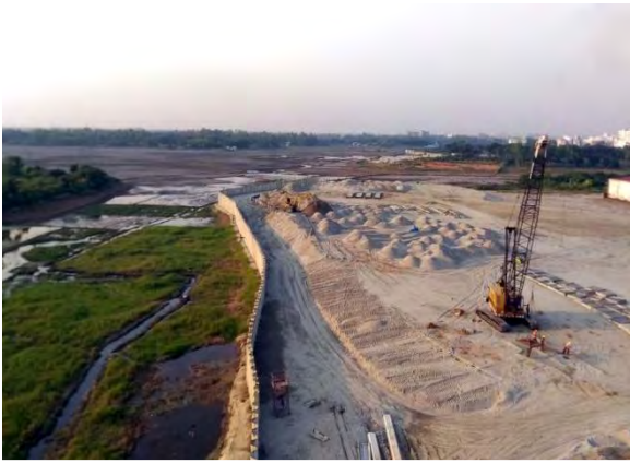
Land Filling & Sheet Pile work at BATB Savar Land Fill Project
