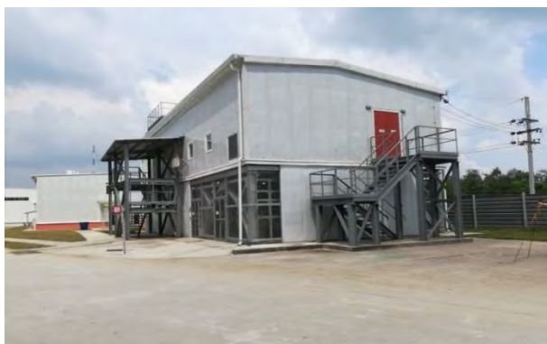
2 storied Steel Building for 33/11 KV Distribution Substation at Rooppur NPP Project, Ishwardi, Pabna
