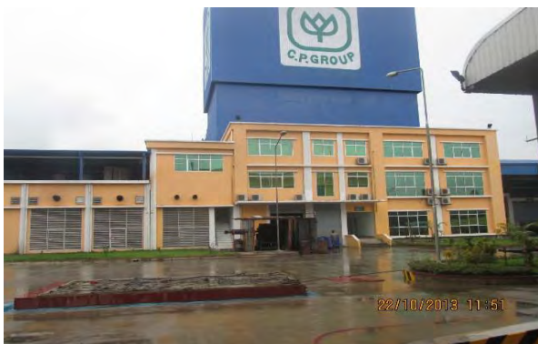
3 Storied Production Building, Total Area: 1950 sqm at C.P Chittagong Feed mill Project, Chittagong.
