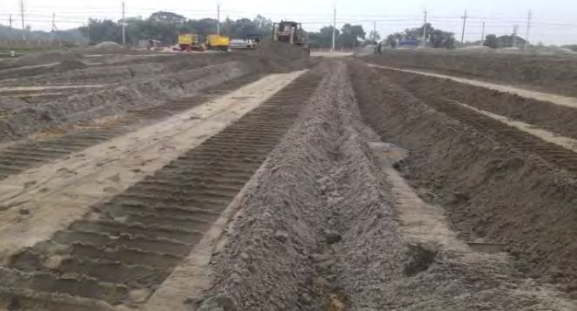
Land Filling work at Trishal Feed Mill Project
