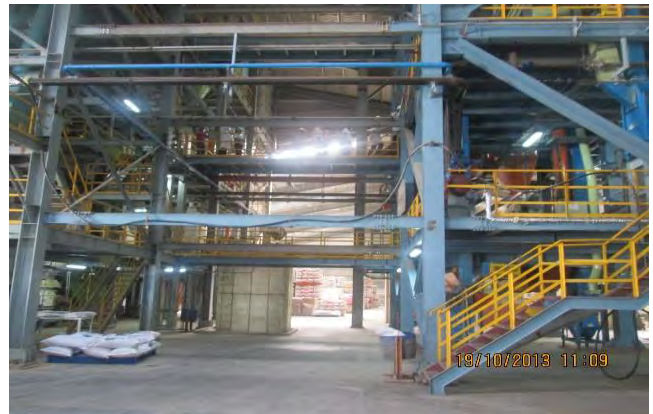
Steel Structure of CP Chittagong Feed Mill Project
