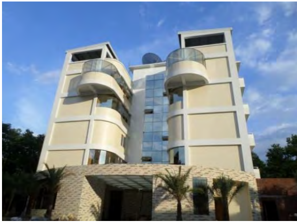
5 Storied Dormitory Building, Total Area: 3500 sqm at C.P Gazipur Feed mill Project, Chandra, Gazipur.
