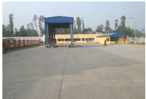
Internal Road/Pavement work at CP Chittagong Feed Mill Project
