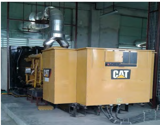
Supply & Installation of 1.2 MVA Generator at CP Bogra Feed Mill Project
