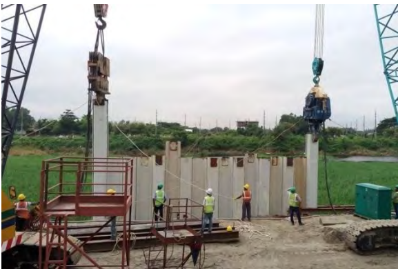
Sheet pile driving work at BATB Savar Land Fill Project
