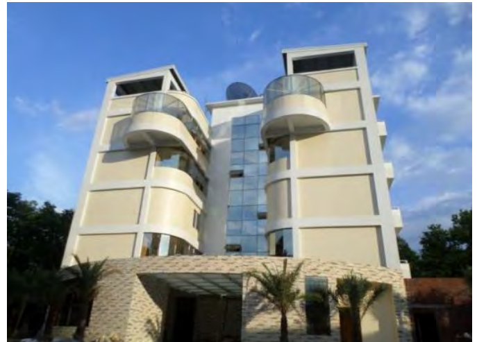
5 Storied Dormitory Building, Total Area: 3500 sqm at C.P Gazipur Feed mill Project, Chandra, Gazipur.
