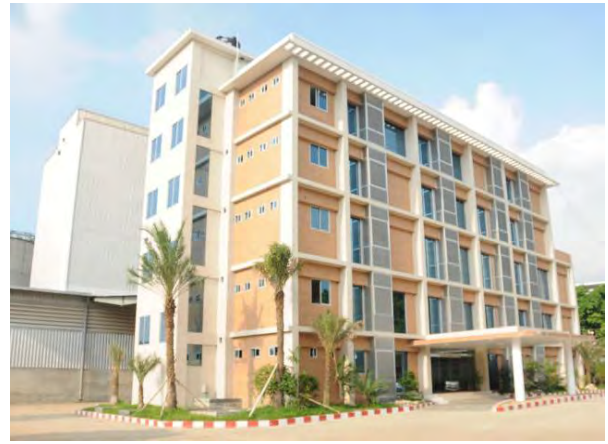
5 Storied Office Building, Total Area: 3500 sqm at C.P Gazipur Feed mill Project, Chandra, Gazipur.
