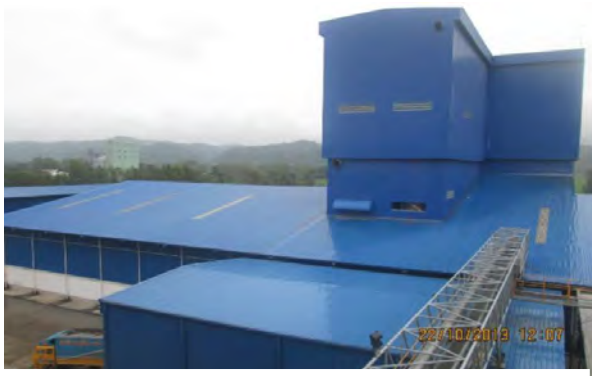
Steel Building of Fish Feed Mill at CP Chittagong Feed Mill Project, Mirsarai, Chittagong.
